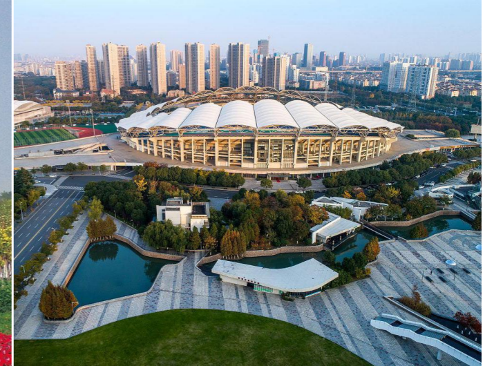
Jiangsu Kunshan Stadium
