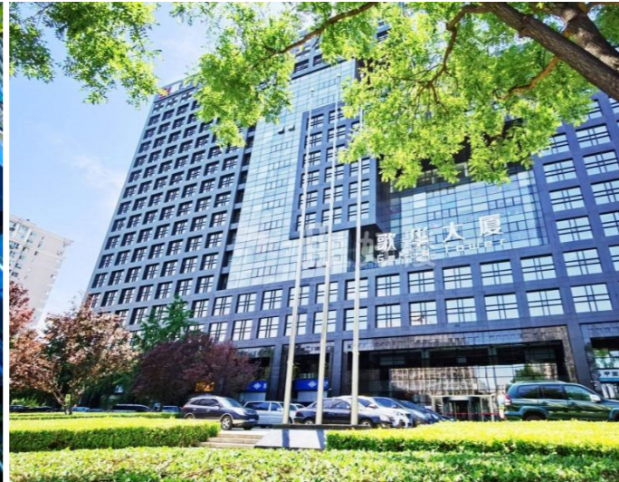
Beijing Gehua Tower
